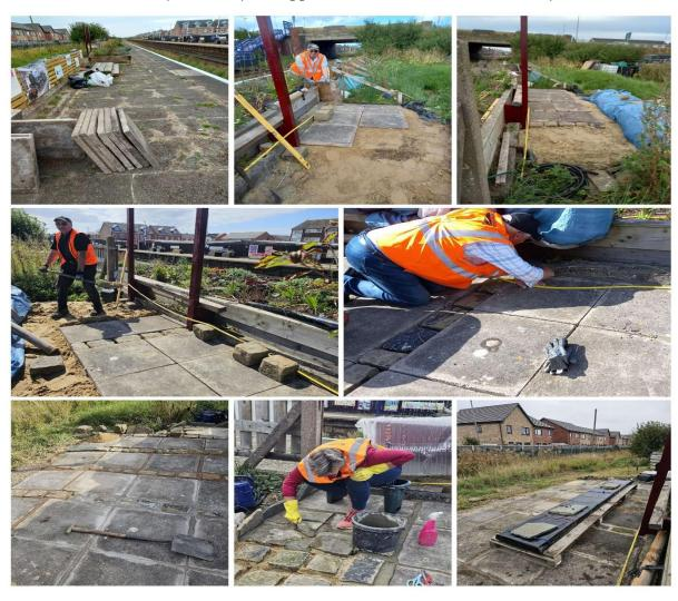
Thankfully we had obtained over 30 paving slabs and stone setts from various local sources at no cost to us and we had previously laid over 1.7 tons of grit sand in late 2023 on top of two layers of membrane to subdue any weeds, but had to order another 800kgs to finish off the paved area. The new station sign is going to be installed in Spring 2025 to coincide with the 200 years of train travel event year.
