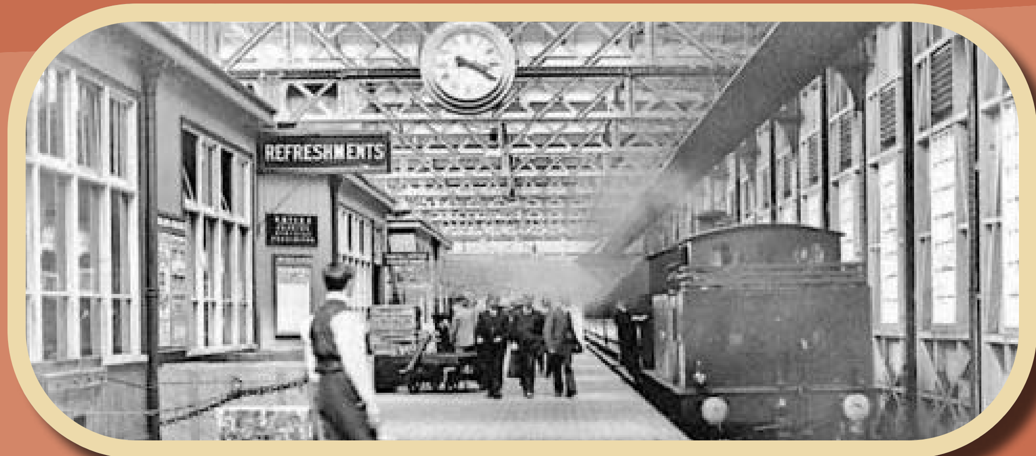
An early atmospheric picture of Heysham Port station shows a busy platform as a steam hauled service arrives.
