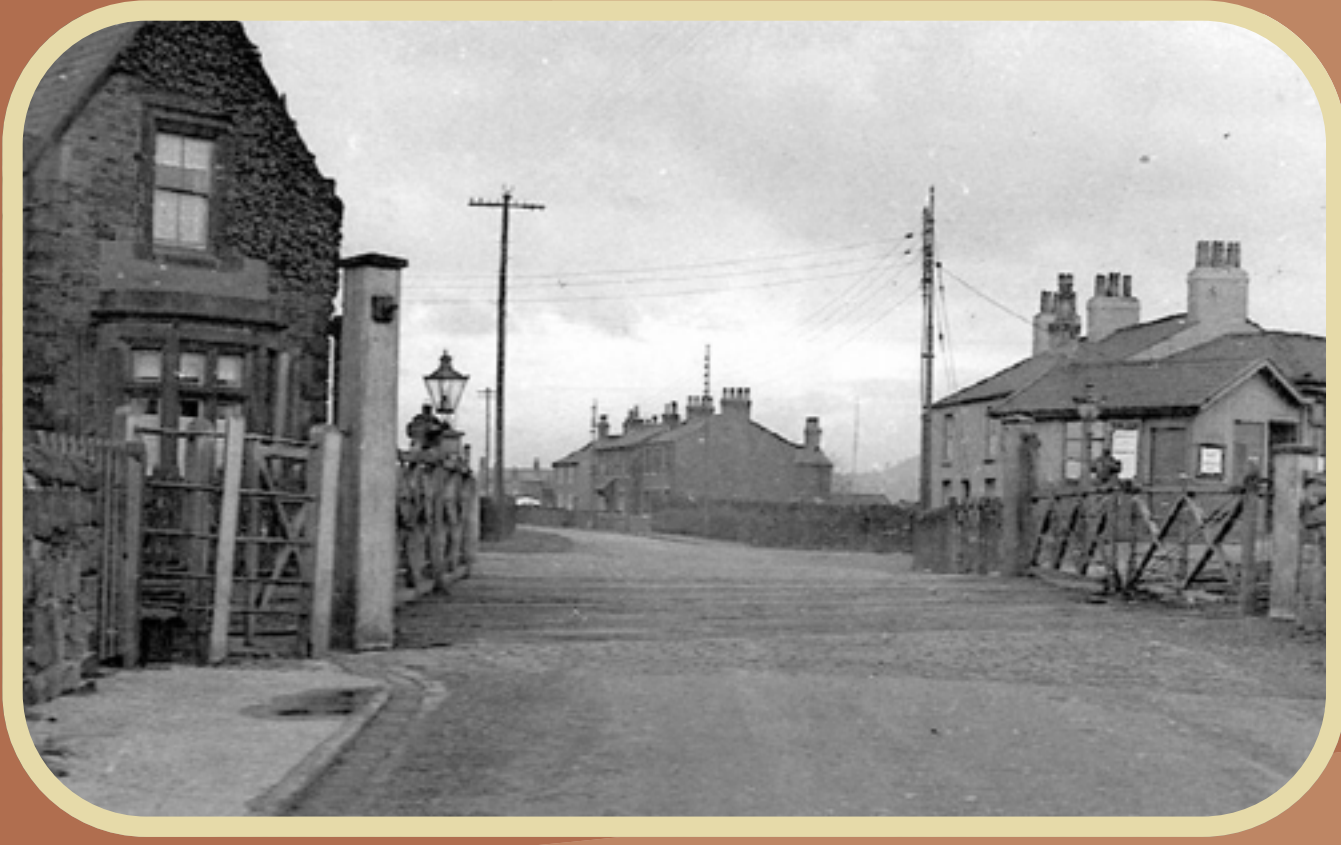
Hoscar crossing looking East
