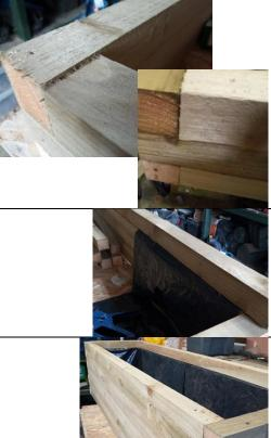
Fix the last layer of timber on top and screw down.
