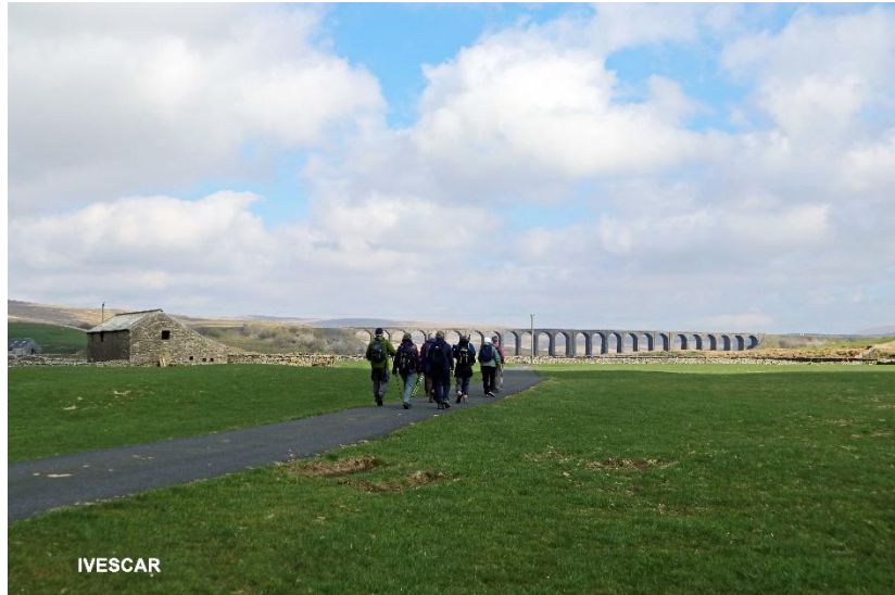
Ribbleshead Viaduct (John Barnes)
