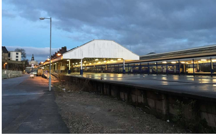
Photograph: Bolton station platform 5.
