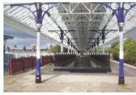
Network Rail has now completed the work to refurbish the canopy at Nelson station and this is now looking resplendent with new colours and new glass in the roof. The track has also been renewed through the station and this completes the work that started with the building of the new bus/rail Interchange. A Friends of Station group has also been formed and
